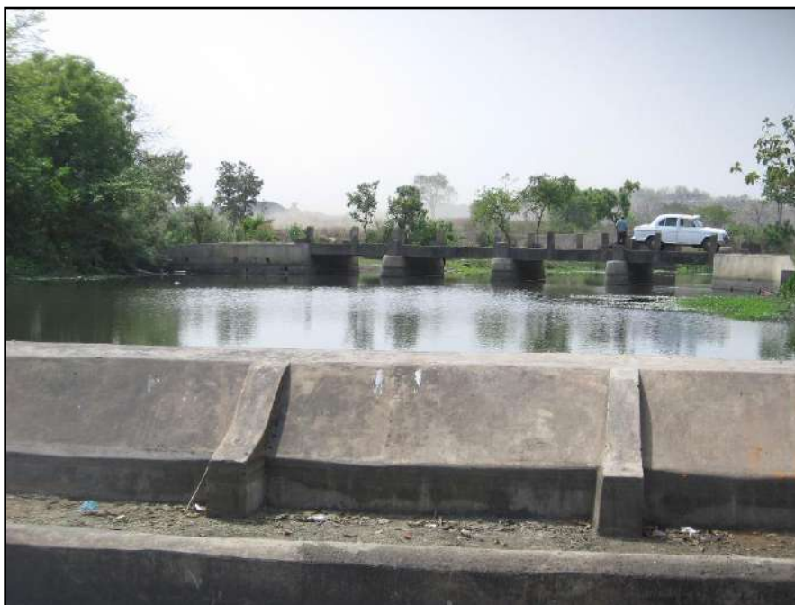
Figure No-2: Check Dams / Nala bunds.
